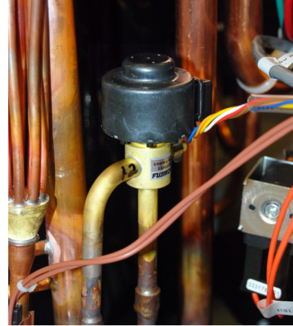
Fig. 1 – Electronic Expansion Valve (EXV)
